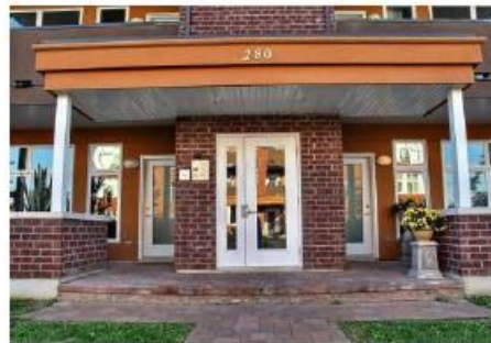
Figure 268 Weather protected entrance
