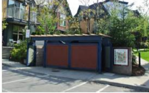
Figure 279 Example of screened waste enclosure
